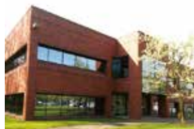
FLIR Systems, Portland
