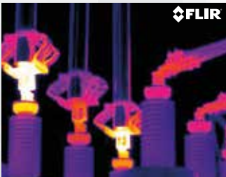
Thermal inspection of a high voltage installation.
