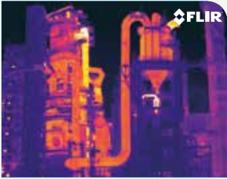
Monitoring a petrochemical installation 24/7 to increase safety.
